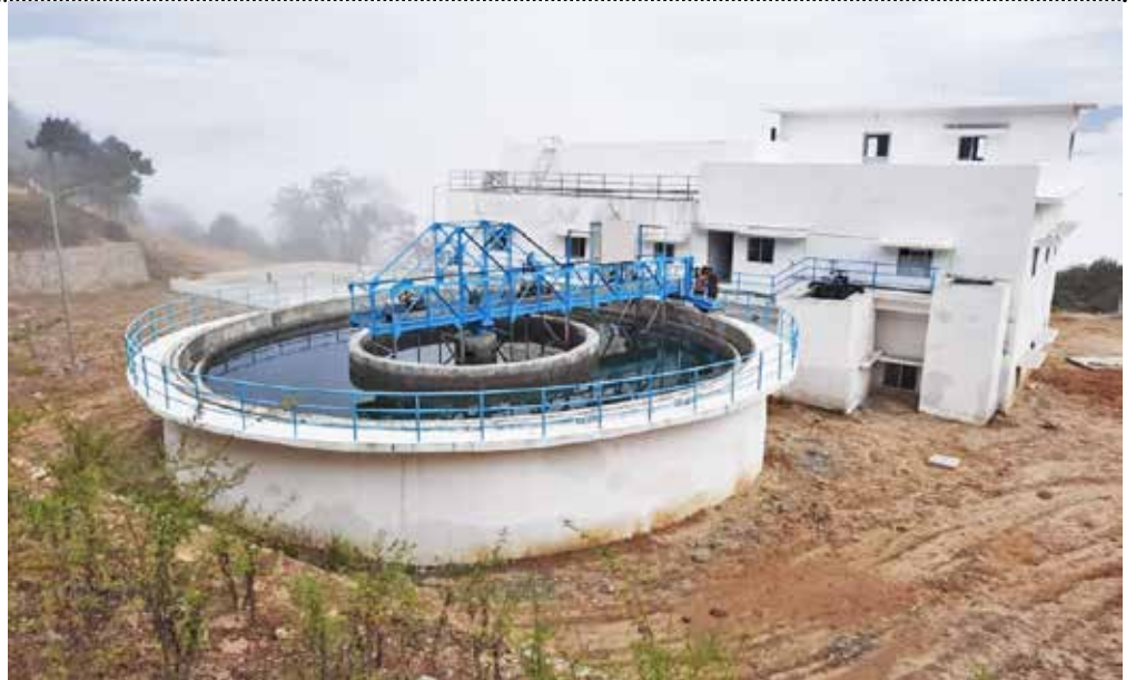
► Water treatment plant constructed in Kanglung, Trashigang
